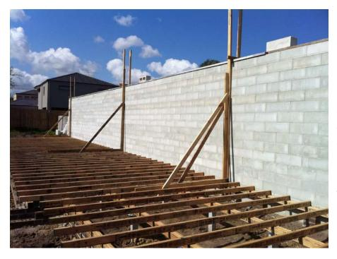
Benex Block walls with returns should be checked for lateral stability. As a rough guide, if a return on a wall is less than 600mm then that end of the wall is without adequate lateral support and requires fixing to a support or bracing.
